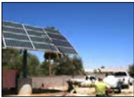
SOLAR PANEL CLEANING
