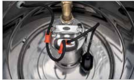
Submersible stainless steel pump for oil discharge
